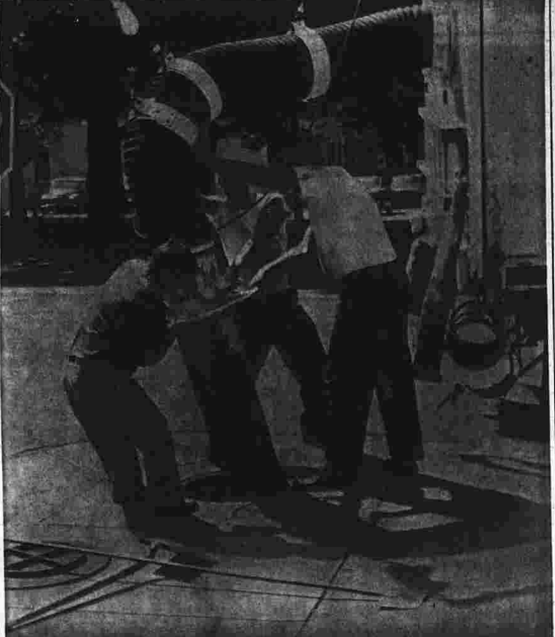
Vacuum Used to Clean Sewers
